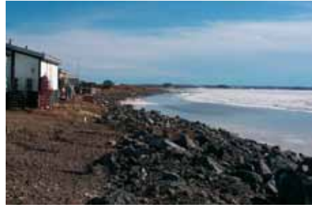
To try and prevent further erosion of the shoreline a wide band of rocks had been put in place.
