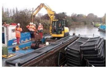
The floating nature of the system, and the ability for water to flow smoothly underneath were important features for the approval of the Environmental Agency (EA) in the flood prone location.
