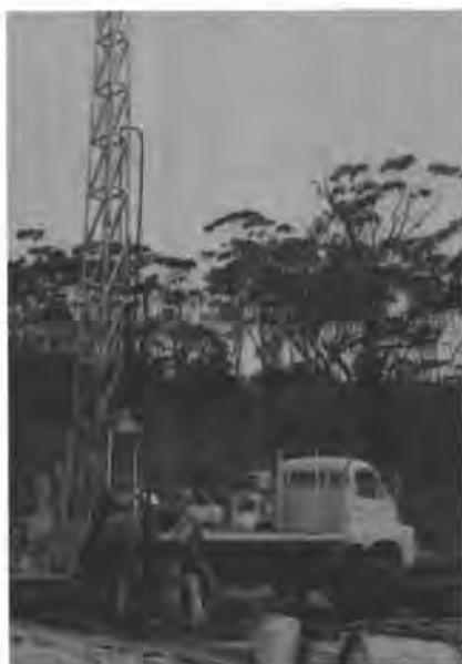
Percussion drill on dry lake bed, drilling a test bore
