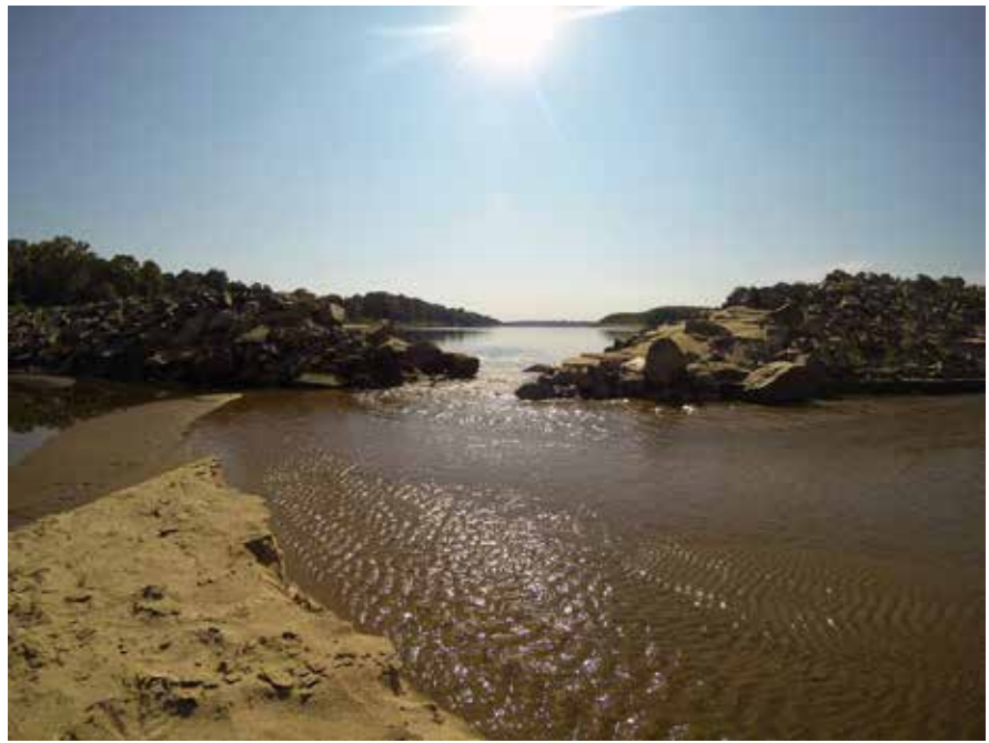
Figure 4 – A dike notch at the Shipland Wildlife Management Area maintains connectivity between the secondary channel and the river. Photograph by Bruce Reid, LMRCC.
