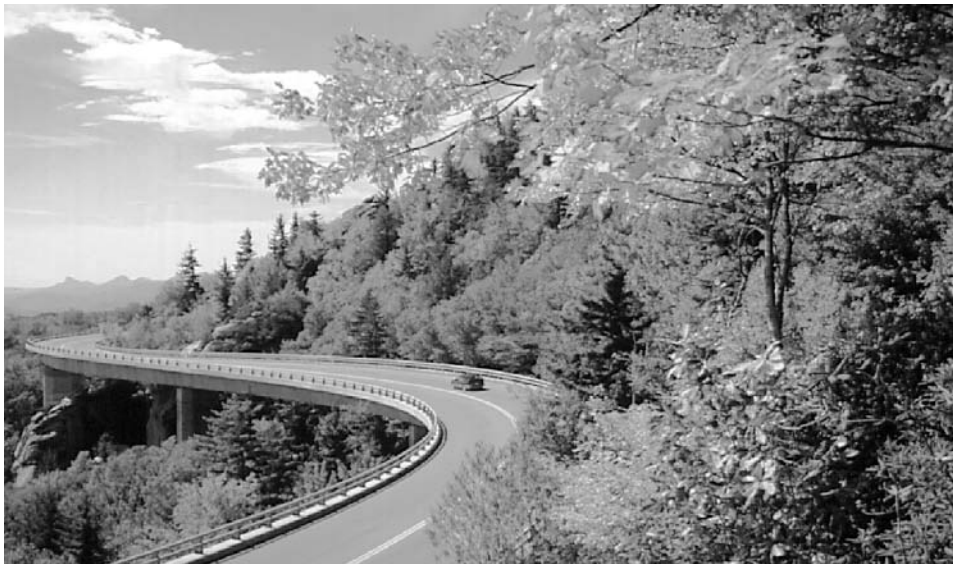
A car on the Blue Ridge Parkway viaduct on Grandfather Mountain. (Photo by Randy Johnson.)
