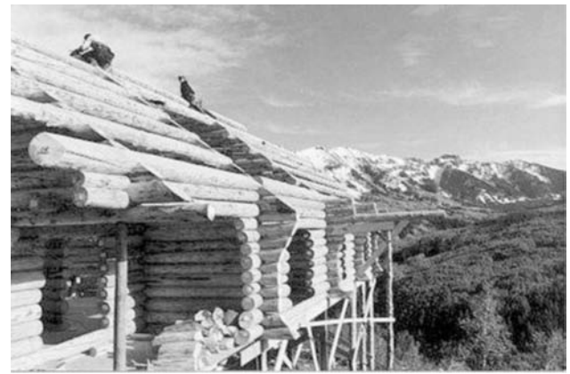
Figure 2—Workers construct an inholder's cabin, which is visible for several miles throughout the West Elk Wilderness, Colorado. Photo courtesy of The Wilderness Land Trust.
