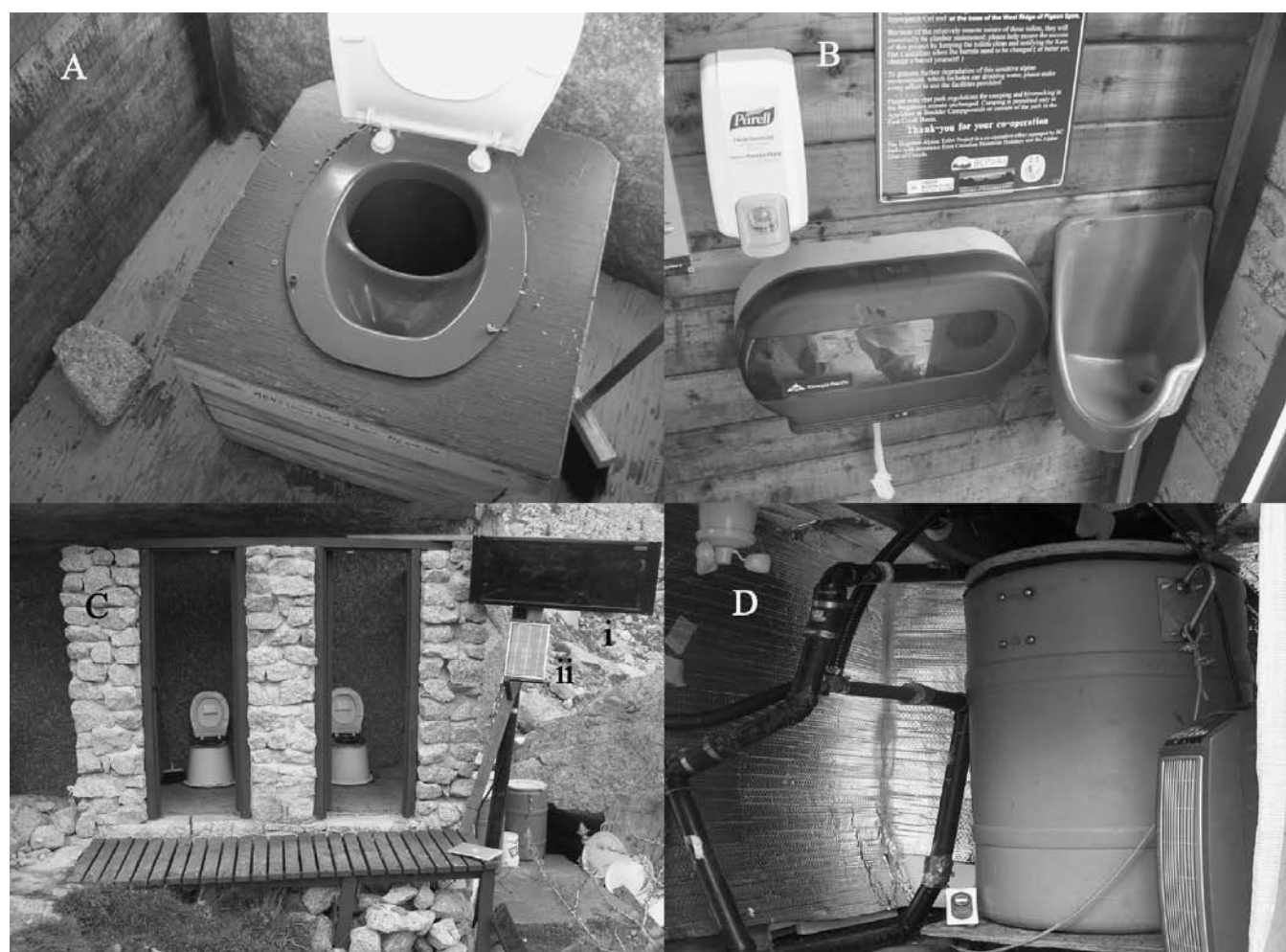
Figure 1 – Alternative toilet waste management treatments at Kain Hut, Bugaboo Park, BC Canada. (A) Urine diversion toilet seat. (B) Urinal with 1-inch braided drain pipe to collection barrel. (C) Lower toilets with UD12V solar hot-air panel (i) above a 5W PV panel (ii). (D) Upper Kain Hut toilet insulated basement, 110V heater, and 110CFM exhaust fan positioned around a 200 L plastic barrel with double garbage bags to collect solids.
