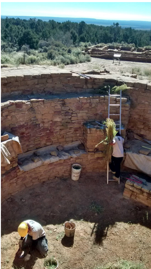
Figure 3 – Southwest Conservation Corps and National Park Ancestral Lands crew completing restoration work on ancient Pueblo kiva.
