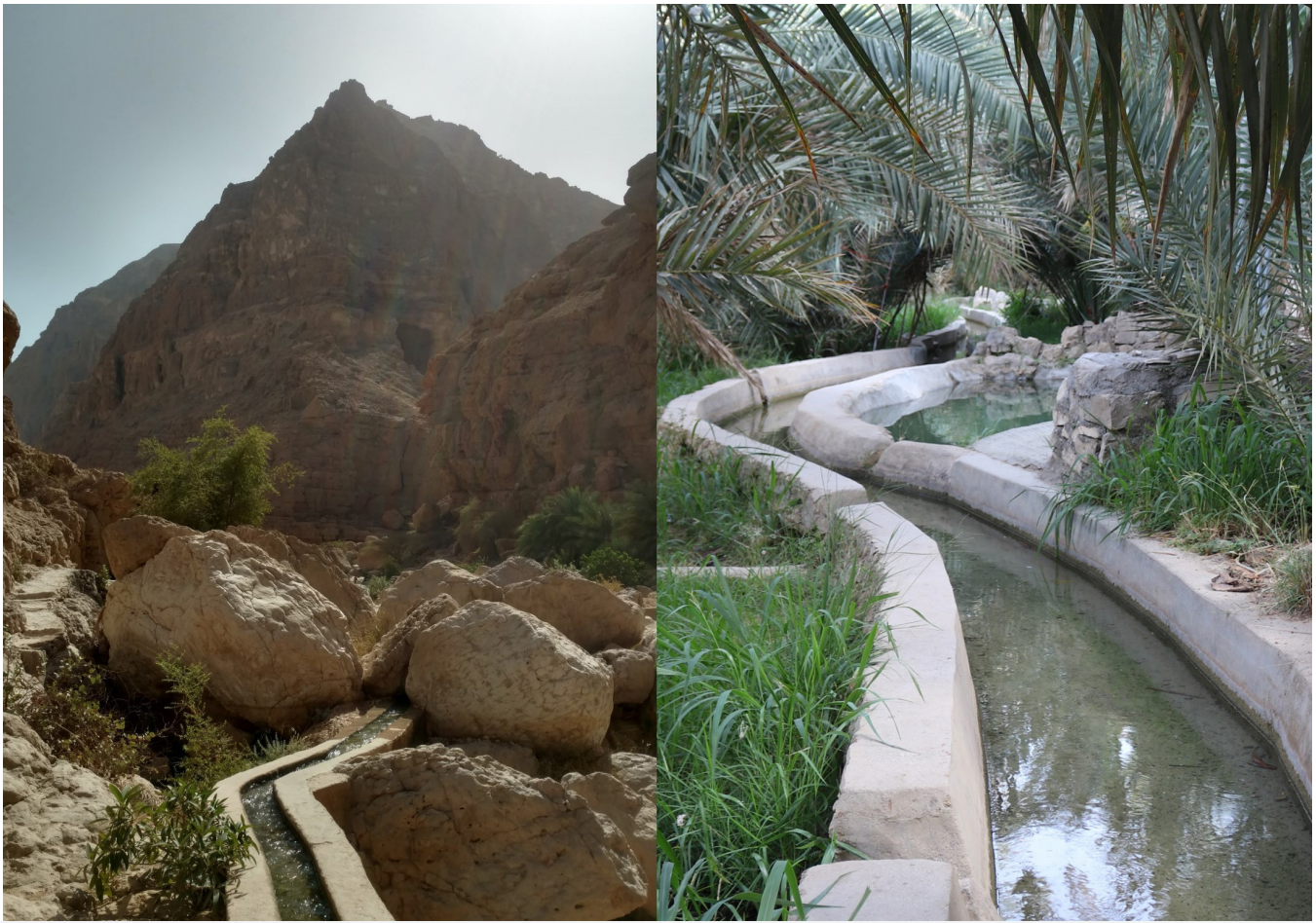
Figure 2 – Examples of falaj irrigation channels in a wadi near the source of the water (left) and within a cultivated area of date palms, fodder grasses, and citrus trees (right).
